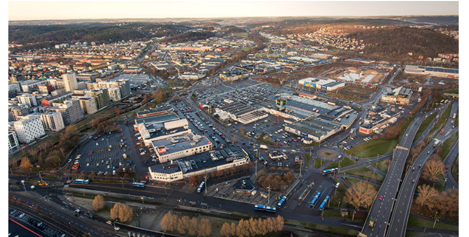
Fig.8: Aerial photo over Kvillebäcken area (current situation)
