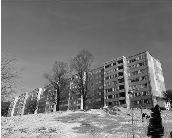
Figure 2: Housing Block at Siriusgatan
